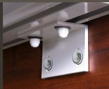
Reveal Bracket Mounting
